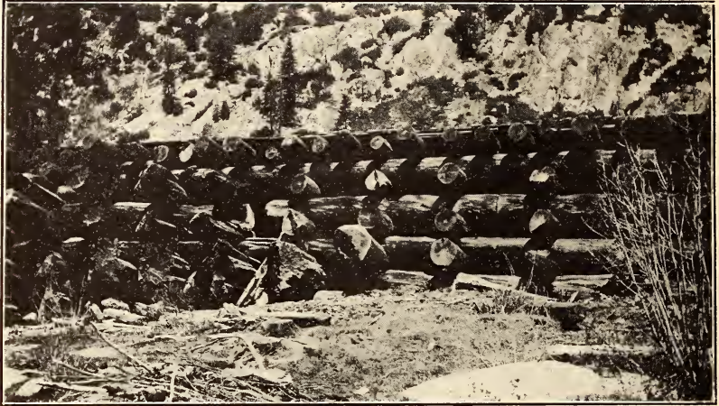
FIG. 5.—Middle Dam, South Fork Stanislaus River, Cal., showing manner of laying logs from the reservoir site. The site was not thoroughly cleared, however, only the best timber suitable for the construction of the dam being used. This standing timber is rotting at the water's edge and
